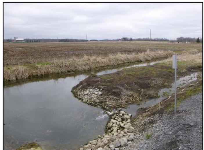
An example of mixed modifications on a headwater drainage feature: dredging and channel hardening with rip rap on Fourth Line Road
