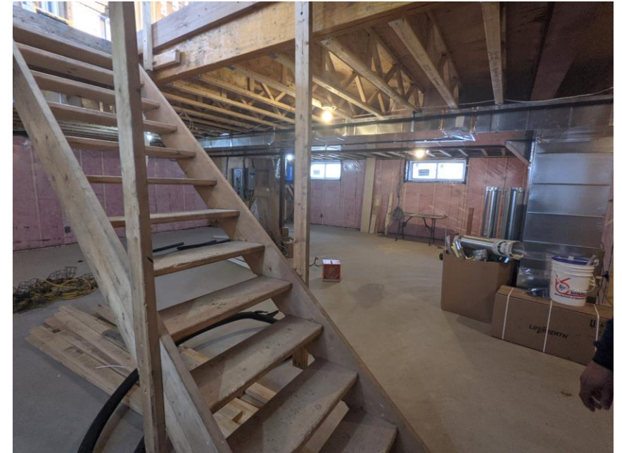
Site Photo: (taken by E. Lalande Oct 12, 2023) showing basement
