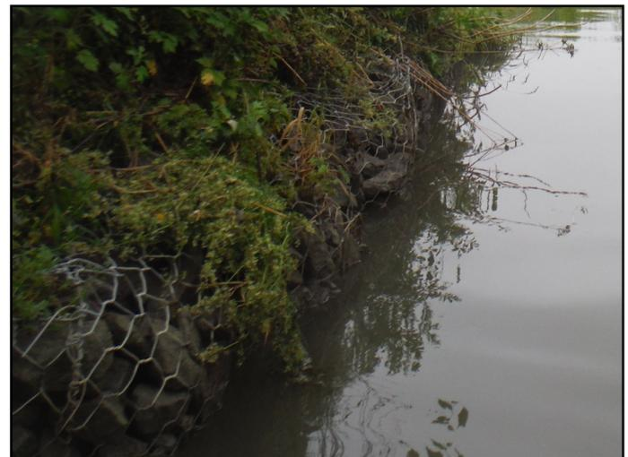
Erosion control measures (ie. gabion baskets) along McEwan Creek
