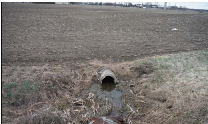
Substantial sediment deposition observed on Malakoff Road
