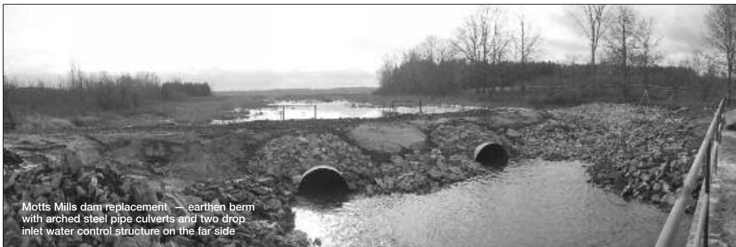
Motts Mills dam replacement — earthen berm with arched steel pipe culverts and two drop inlet water control structure on the far side
