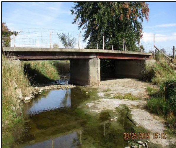
500 Beckwith 9 Line (Upstream)
