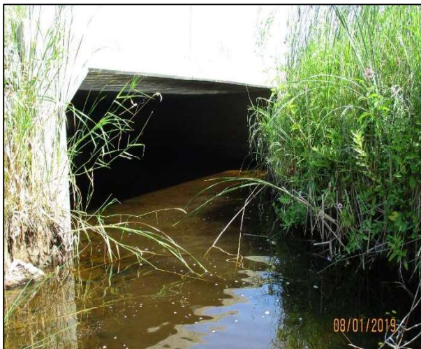
Richmond Rd Culvert (Upstream)
