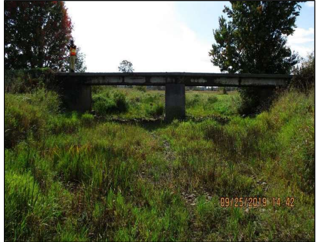
442 Beckwith 9 Line (Downstream)
