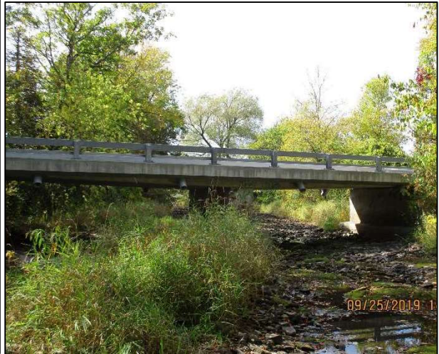
McCafferey Trail Bridge (Downstream)
