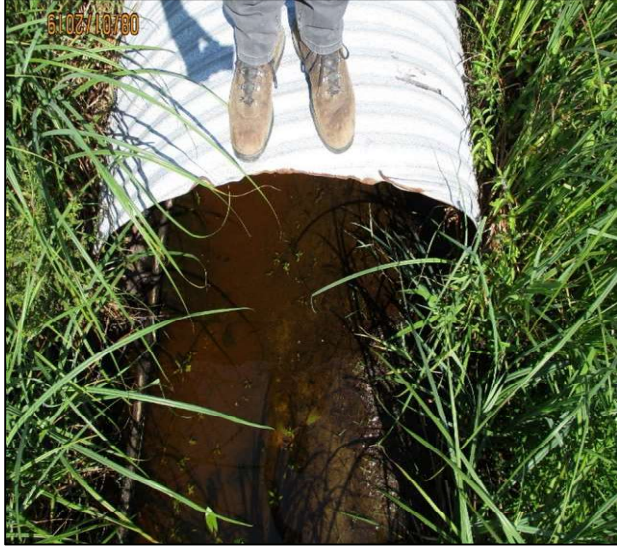
Franktown Swamp Culvert (Upstream)
