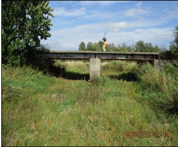
442 Beckwith 9 Line (Upstream)
