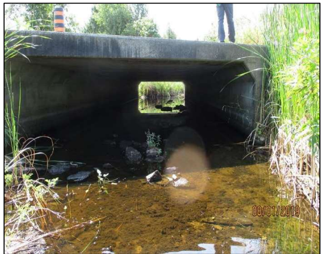
Richmond Rd Culvert (Downstream)
