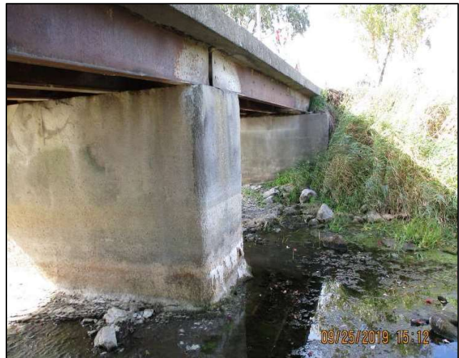
500 Beckwith 9 Line (Downstream)
