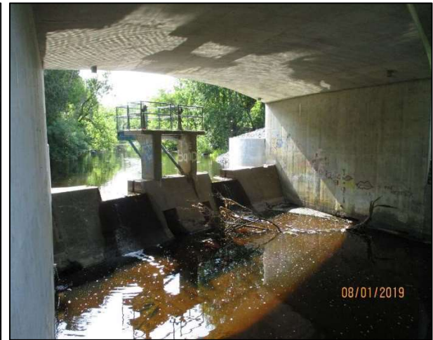
Ashton Station Dam (Downstream)
