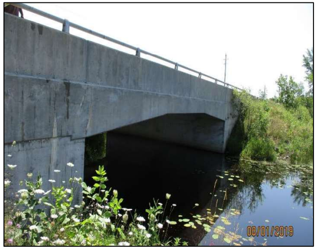
Beckwith 9 Line Bridge (Downstream)
