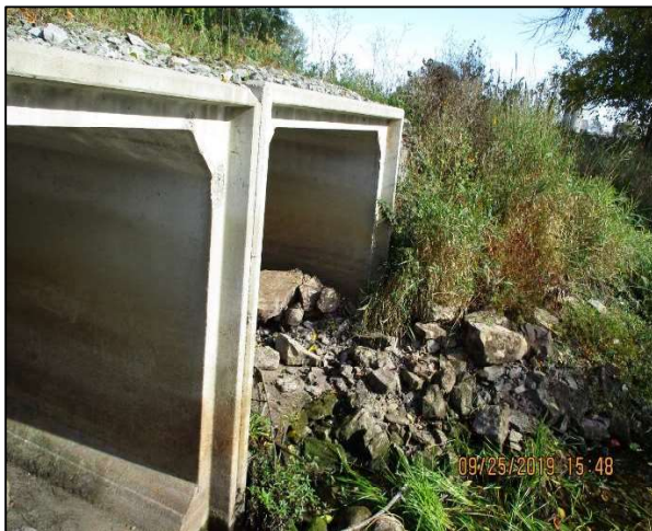
562 Beckwith 9 Line (Upstream)
