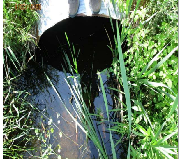
Franktown Swamp Culvert (Downstream)
