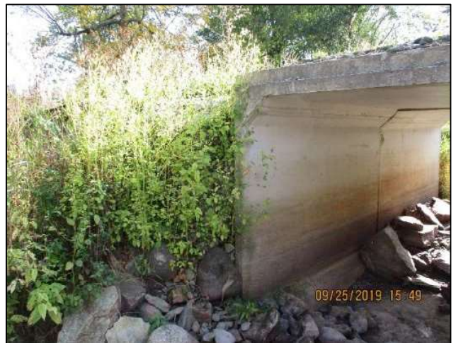
562 Beckwith 9 Line (Downstream)
