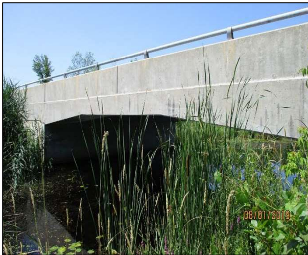
Beckwith 9 Line Bridge (Upstream)
