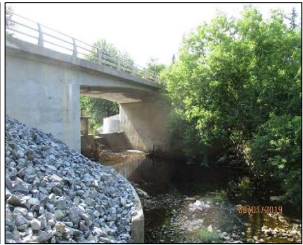
Ashton Station Bridge (Downstream)
