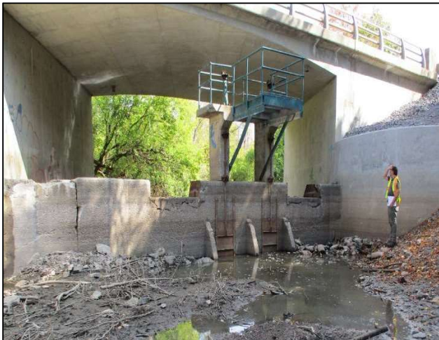
Ashton Station Dam (Upstream)
