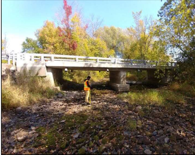
McCafferey Trail Bridge (Upstream)
