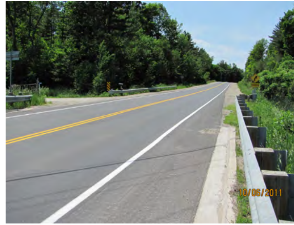
Rideau Ferry Road (looking west)
