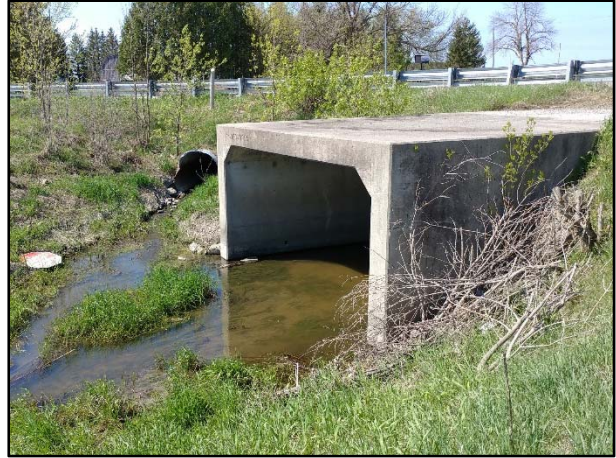
Century Road at 3 rd Line Road (Downstream)
