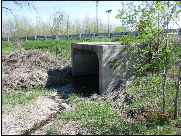
Century Road at 3 rd Line Road (Upstream)
