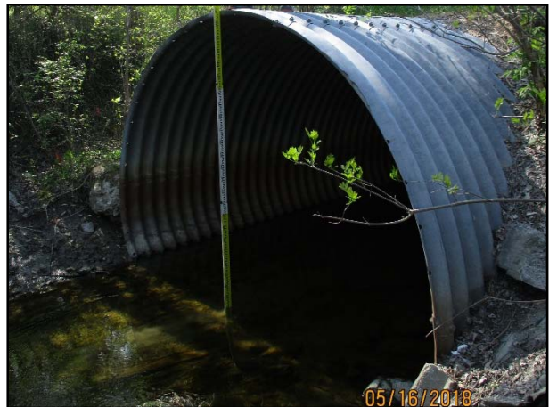
3 rd Line Road (Downstream)
