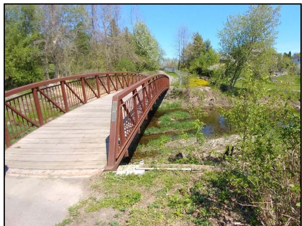
Revell Pedestrian Bridge (Upstream)
