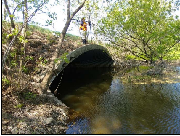
Century Road west of 1 st Line (Upstream)
