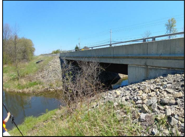
Bankfield Road (Downstream)
