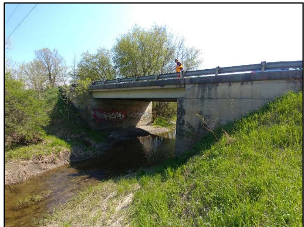
2 nd Line Road (Downstream)
