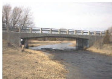
File : Aut_3059.jpg Description: Downstream side of bridge
