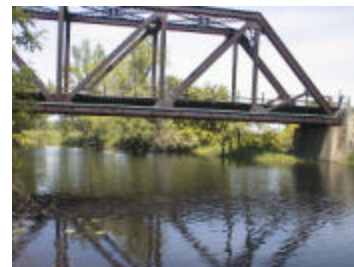
File : Aut_3395.jpg Description: Downstream side of bridge
