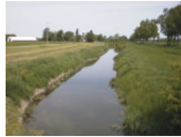
File : Aut_33907.jpg Description: Looking D/S
