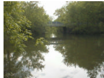
File : Aut_3375.jpg Description: Downstream side of bridge
