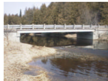
File : Aut_3102.jpg Description: Downstream side of bridge
