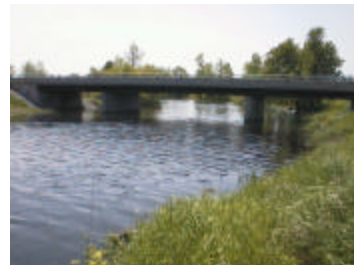
File : Aut_3408.jpg Description: Downstream side of bridge
