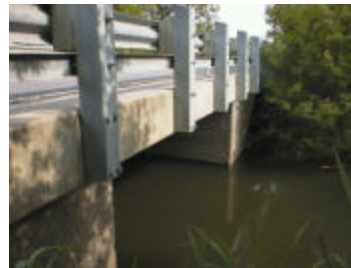
File : Aut_3376.jpg Description: Upstream side of bridge
