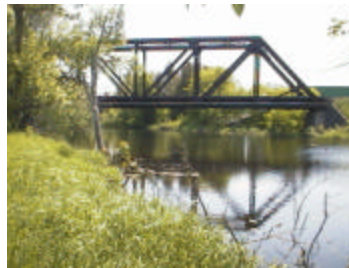
File : Aut_3397.jpg Description: Upstream side of bridge
