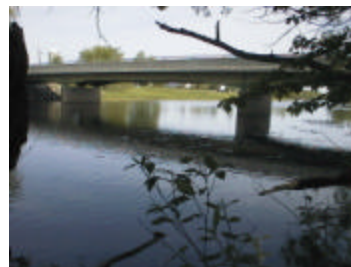
File : Aut_3381.jpg Description: Upstream side of bridge
