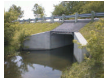
File : Aut_3391.jpg Description: Downstream side of culvert
