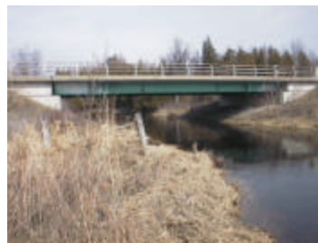
File : Aut_3058.jpg Description: Upstream side of bridge
