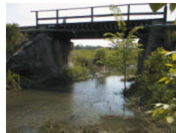
File : Aut_3385.jpg Description: Downstream side of bridge
