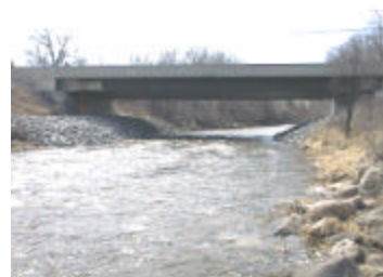
File : Aut_3009.jpg Description: Downstream side of bridge
