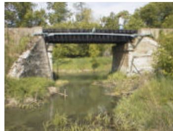
File : Aut_3384.jpg Description: Upstream side of bridge
