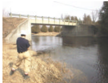
File : Aut_3065.jpg Description: Upstream side of bridge
