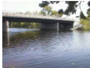
File : Aut_3403.jpg Description: Upstream side of bridge
