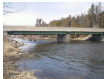
File : Aut_3014.jpg Description: Downstream side of bridge
