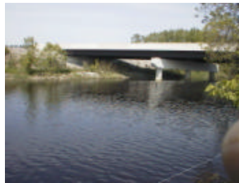
File : Aut_3415.jpg Description: Upstream side of bridge
