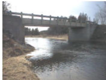
File : Aut_3066.jpg Description: Downstream side of bridge
