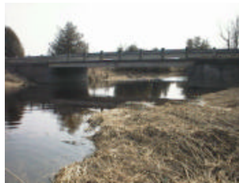
File : Aut_3105.jpg Description: Upstream side of bridge
