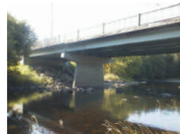
File : Description: Downstream side of bridge
