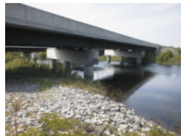
File : Aut_3411.jpg Description: Downstream side of bridge
