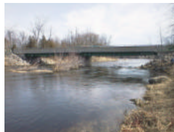
File : Aut_3013.jpg Description: Upstream side of bridge
