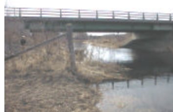
File : Aut_3055.jpg Description: Downstream side of bridge
