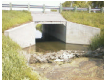
File : Aut_3392.jpg Description: Upstream side of culvert
