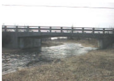
File : Aut_3101.jpg Description: Upstream side of bridge
