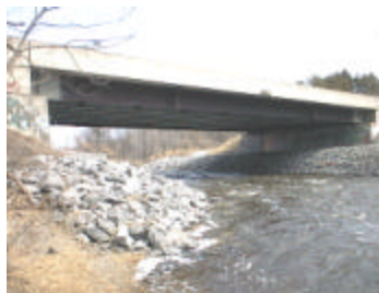
File : Aut_3010.jpg Description: Upstream side of bridge
