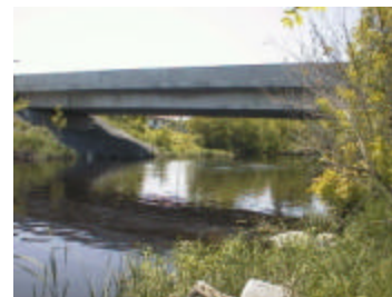
File : Aut_3398.jpg Description: Downstream side of bridge
