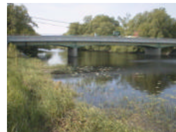
File : Aut_3380.jpg Description: Downstream side of bridge
