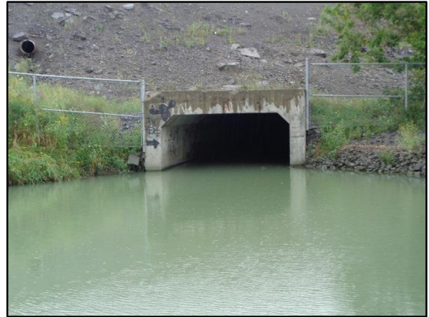
RR174 Queensway (Downstream)
