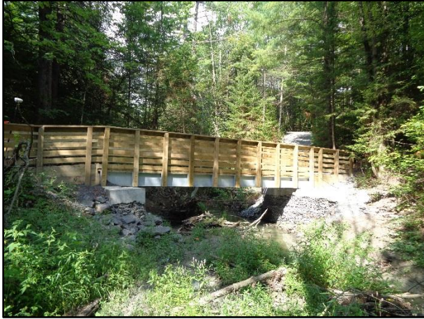
N of Turnberry Pedestrian Bridge (Upstream)
