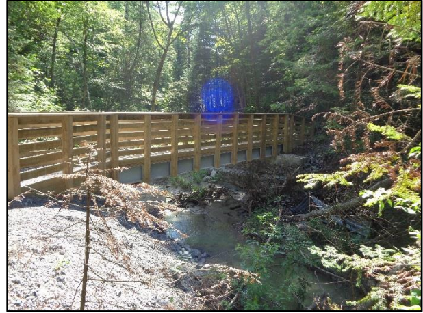
N of Turnberry Pedestrian Bridge (Downstream)
