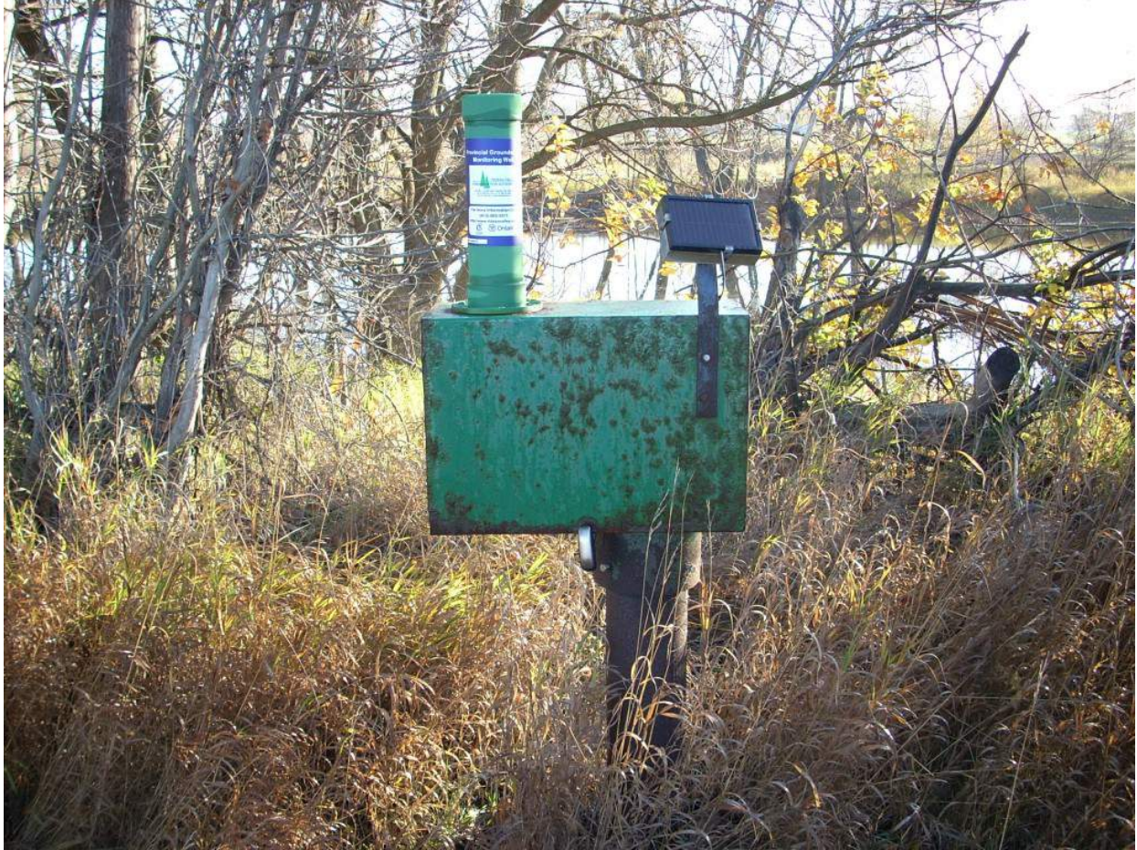
Well- 156-2- Located along the Twin Elm Bridge.
