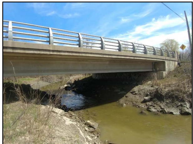
River Road (Downstream)
