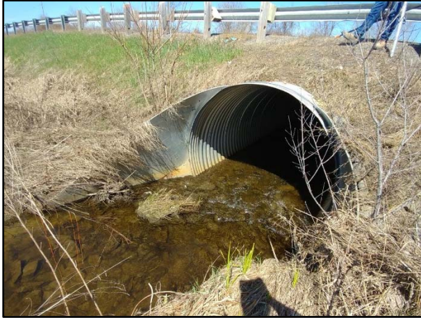
Rideau Road (West of Downey Road) (Upstream)
