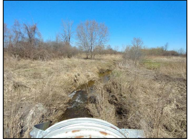
Rideau Road (West of Downey Road) (Downstream)
