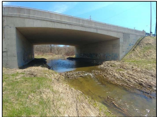
Limebank Road (Downstream)
